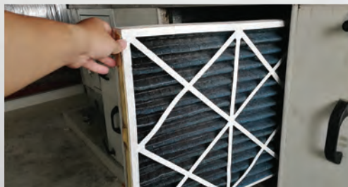
A/C Filter Replacement
