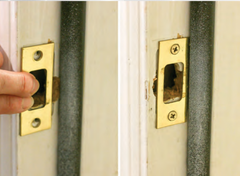
Strike Plates on Door Latch
