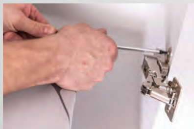
Cabinet-Hinge Repair
