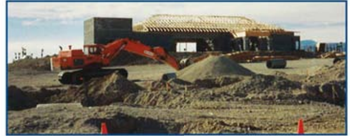
The Vista Grille Under Construction
