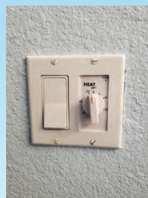
Ceiling heater and control switches
