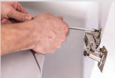
Cabinet-Hinge Repair
