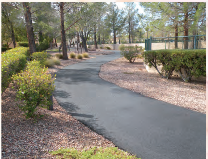
Refurbished walking path at Mountain Shadows.
