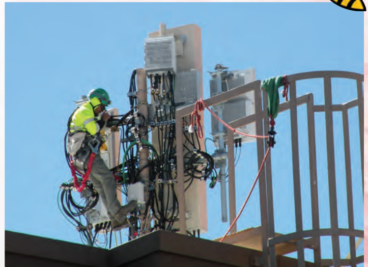
Cell towers are being updated on the Pinnacle roof.
