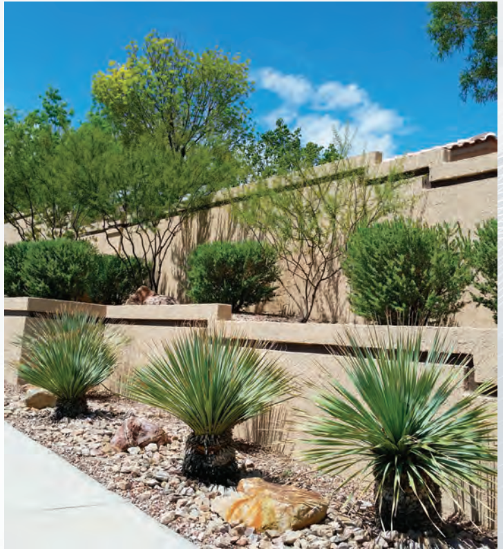
Perimeter walls, which Sun City is responsible for maintaining are constructed of masonry and stucco, and are identified by a brown paint stripe recessed in the walls. In all, Sun City's common walls cover roughly 31 miles of streets throughout the community. Photo by Stu Gershon/Link
