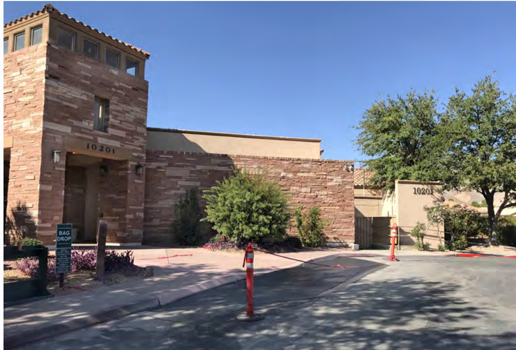
The curb that once extended beyond the sidewalk at the entrance to Highland Fall's clubhouse has been removed to make way for two-car access in the lane. Photo by Jeannette Carrillo/Link.
