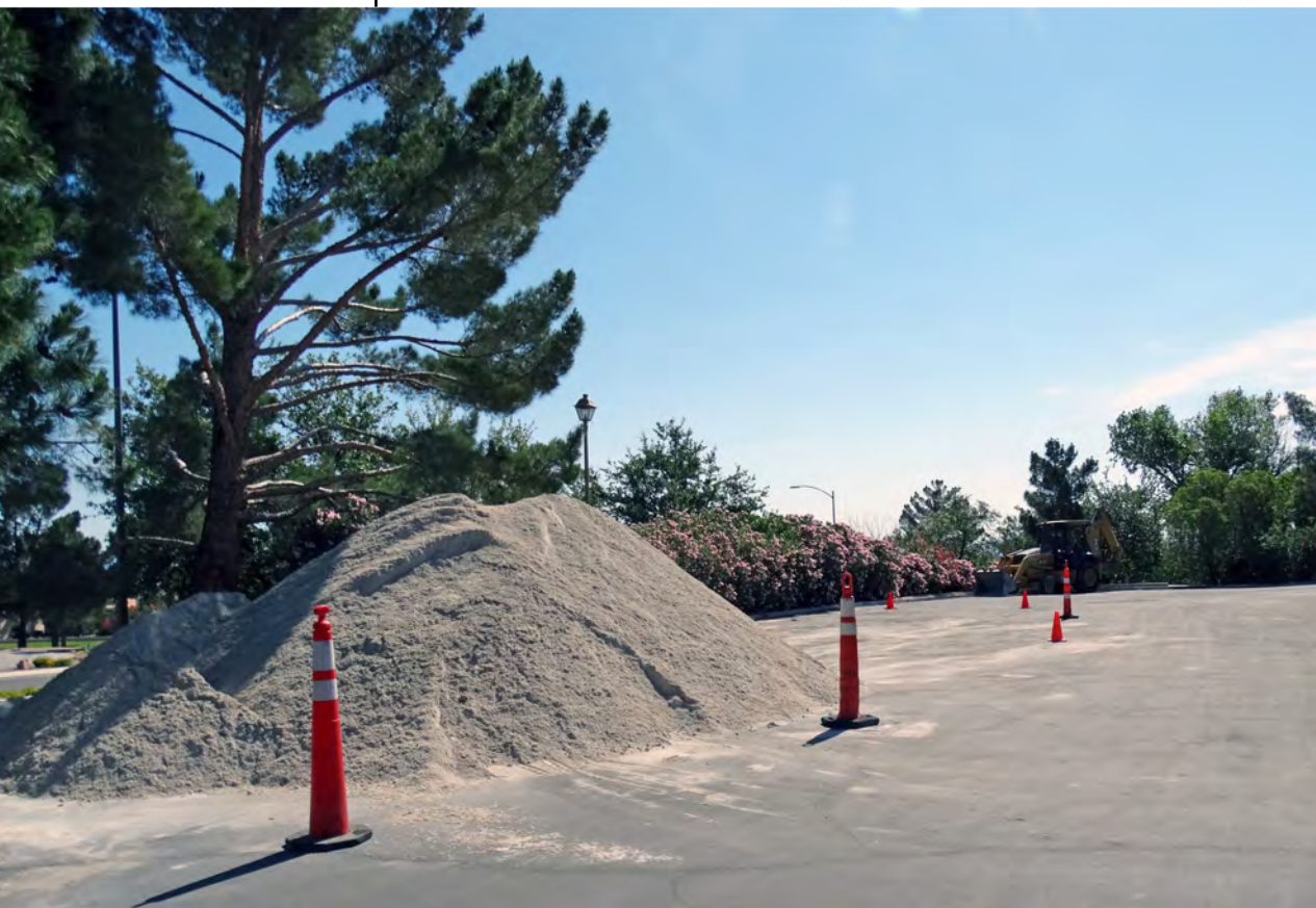
The bunker project has been slowed due to the unavailability of sand. Only a couple of holes remain at Highland Falls, with work on Palm Valley to follow.
